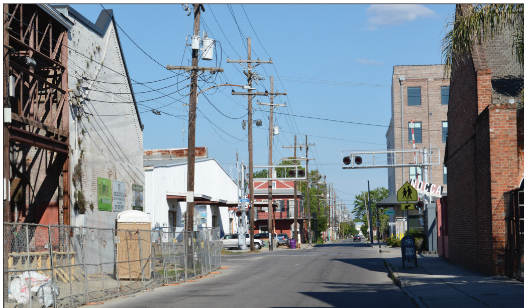
A view of Chartres Street with the existing NOCCA campus on the right and the in-progress adaptive reuse complex on the left.
