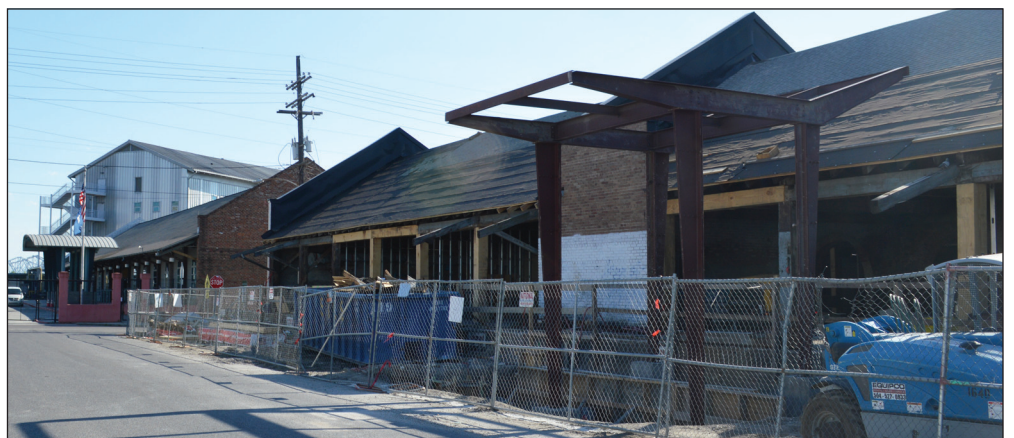
The same view of the new NOCCA complex as is pictured in the rendering above as it looks today. Construction has begun and has an anticipated end date of September 2014.
